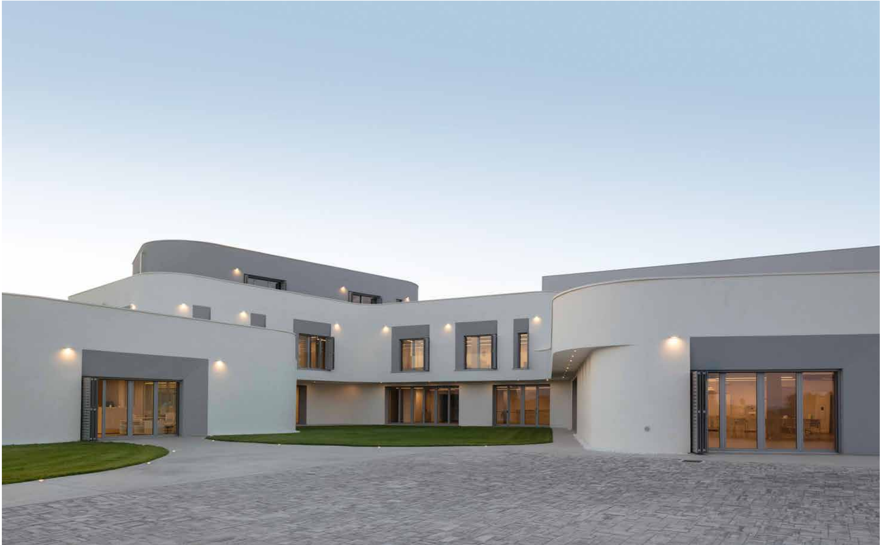
Campus Une, Correggio, Italy. Project: Rizoma Architecture Memento20 Grigio
