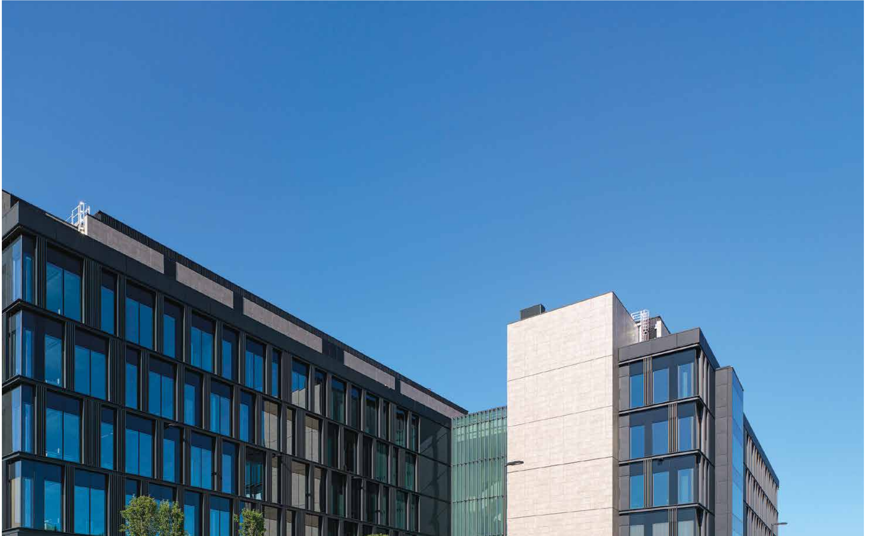
Chiesi Headquarter, Parma, Italy. Project: Project EFA studio di architettura Mstone Gris Fleury
